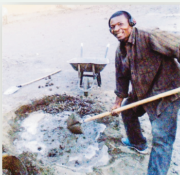
Above: Work in progress on the Youth Center; Bottom: Worker mixing cement
