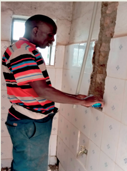
Installation of insulated hot water pipes at Rushoroza Mother House in Kabale, Uganda
