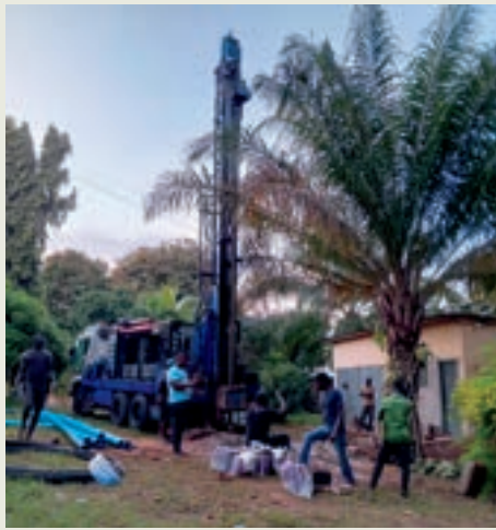
Workers install the new 200-foot well at Collège Notre Dame d'Afrique.
